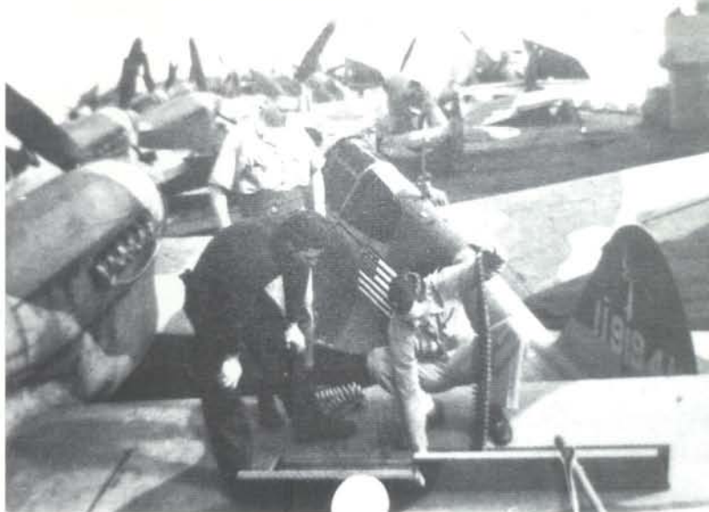
Armors load the .50 caliber wing guns of a P-40F Warhawk of the 325th Fighter Group on the deck of USS RANGER while enroute to North Africa. (Checkertail Clan)
