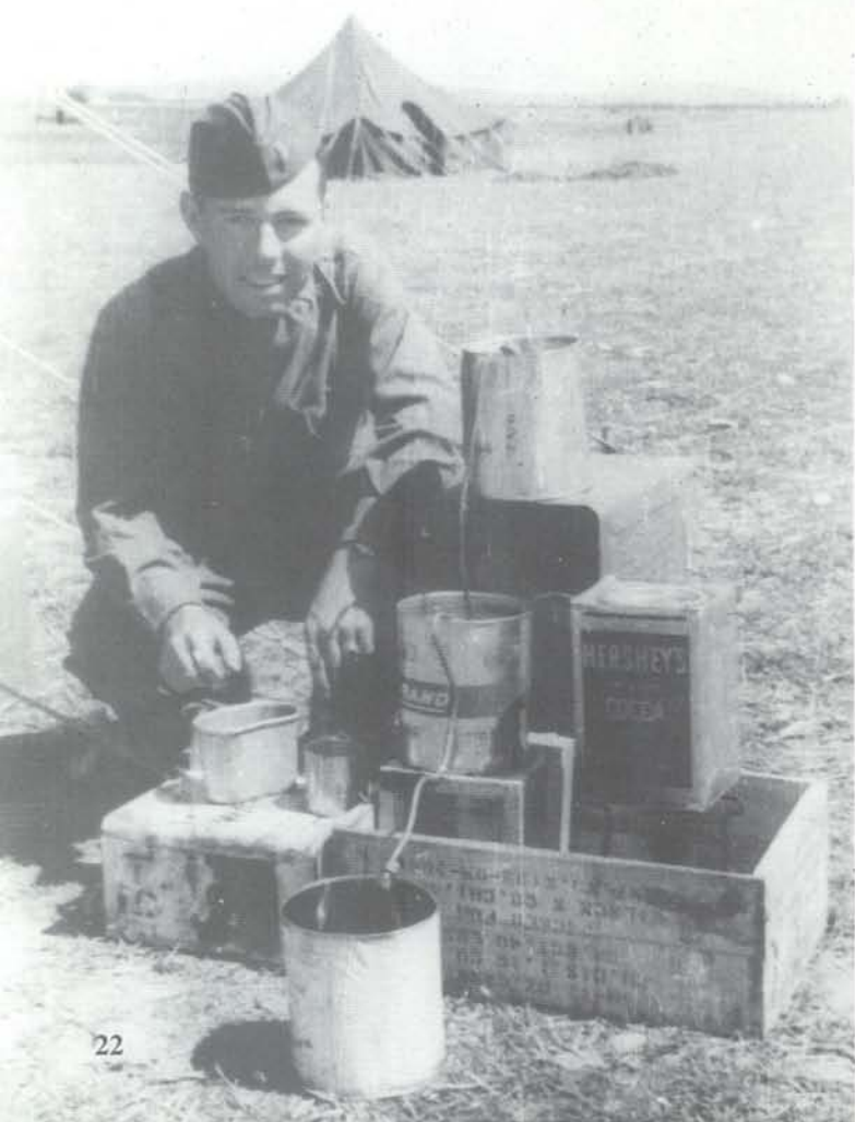
Captain Bunn Hearn looks over the water heater which made the shower a more comfortable and luxurious experience. P-40 belly tanks had more than one use in the desert. (John C. A. Watkins)
